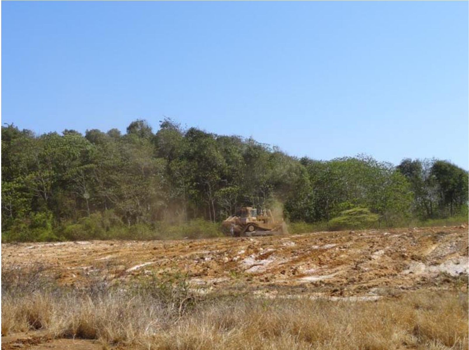
Mining company D9 preparing an old mine site for agriculture
